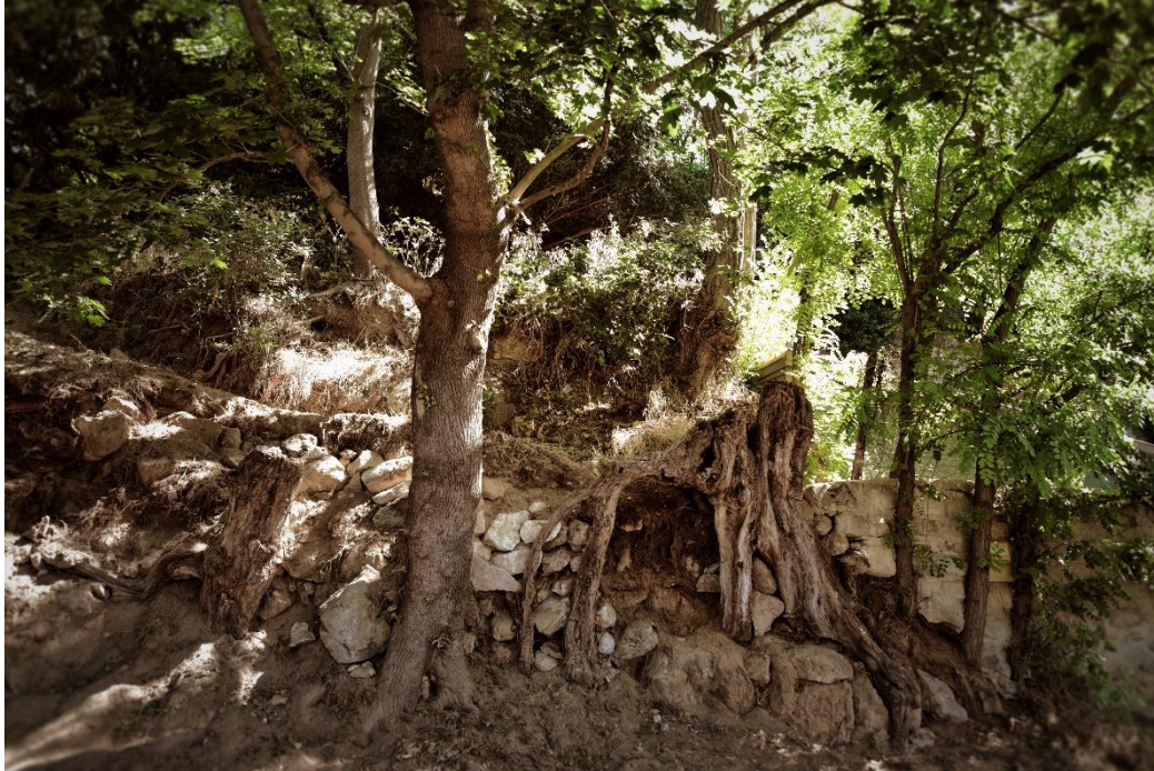
The condition of the hillside in Auvers-sur-Oise on 30 May 2020, ©arthénon
